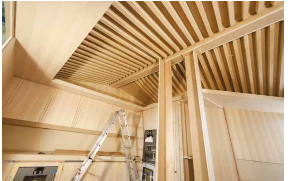
Installation check at our carpenter laboratory
